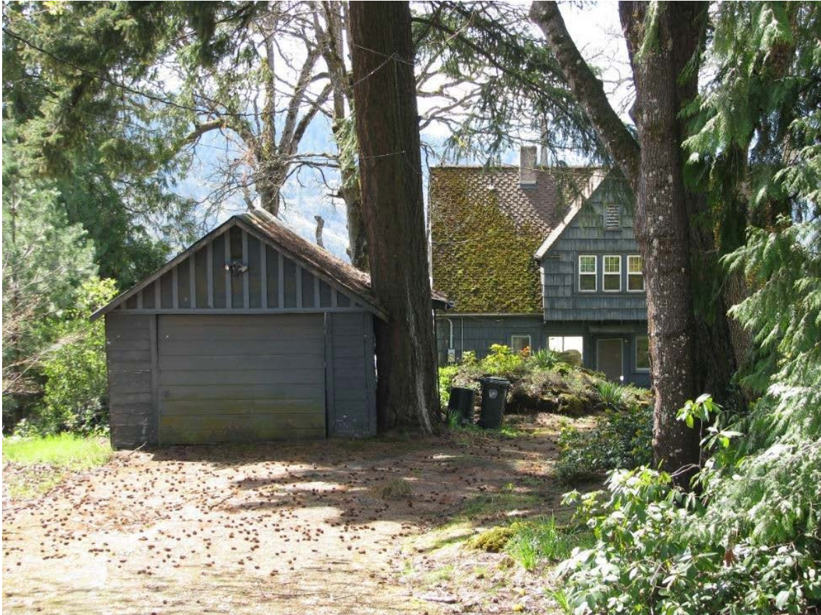
Figure 4. 301 SE Oak Street, looking southwest towards Hood River Bridge.
