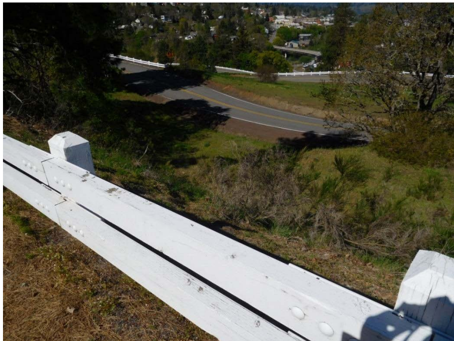
Figure 4. Detail of loops' elevation change and railing. Looking west.
