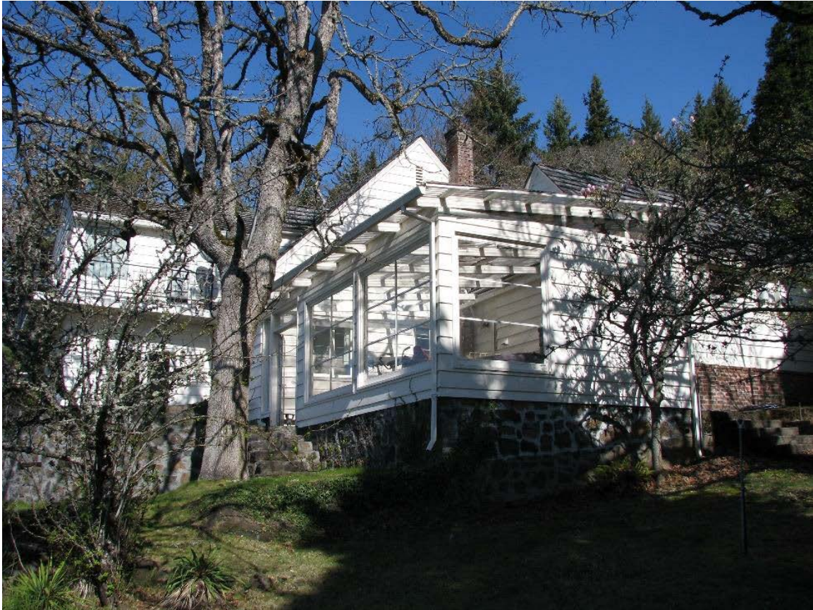
Figure 5. 447 W Jewett Boulevard south elevation and enclosed patio, looking northwest.
