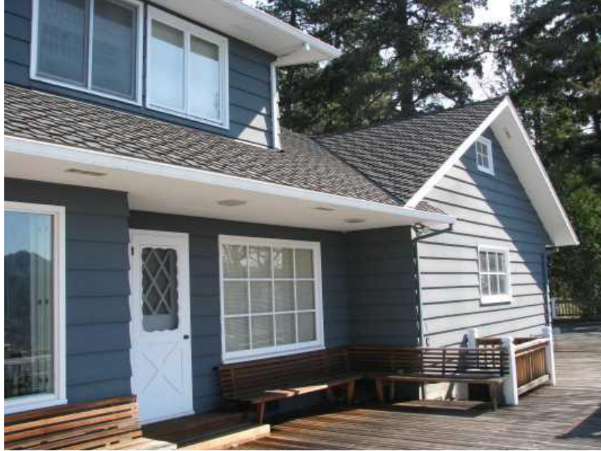
Figure 6-9. Ranch-style residence at 435 W Jewett Boulevard/Van Alstine House (1965) in White Salmon, Washington
