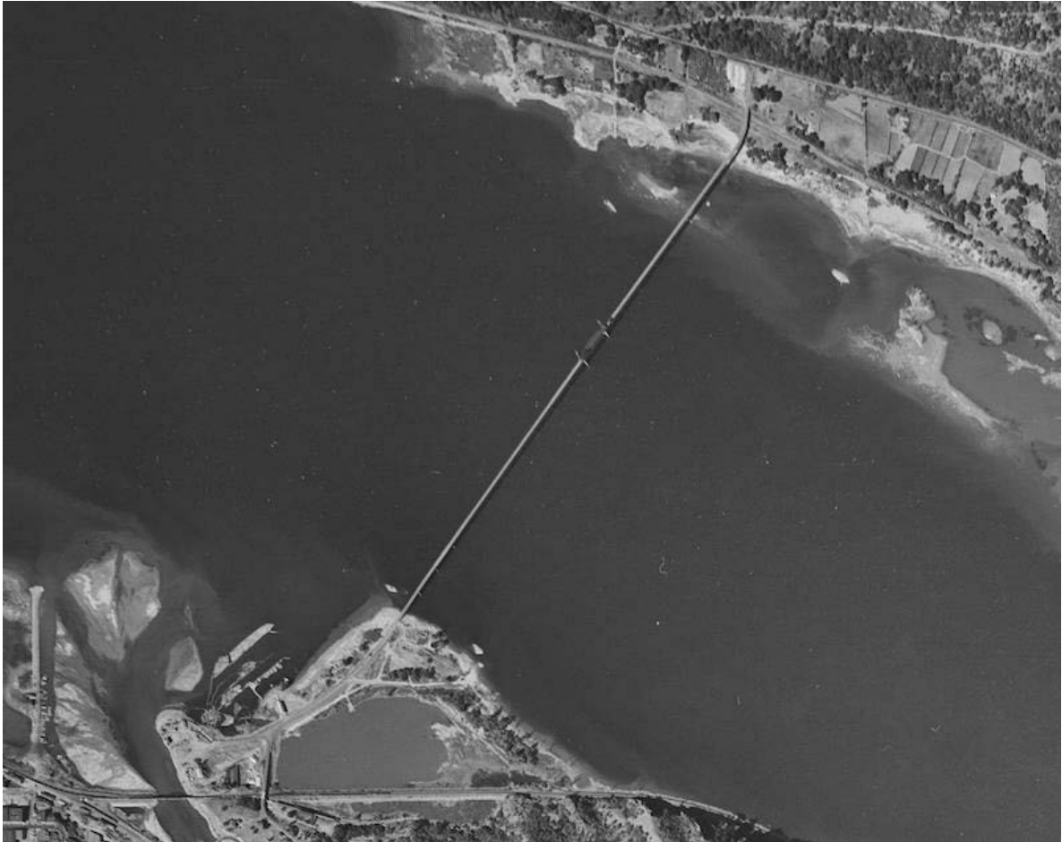
Figure 4. Aerial photograph dated 1947 depicting the Hood River Bridge (Courtesy of earthexplorer.usgs.gov .)
