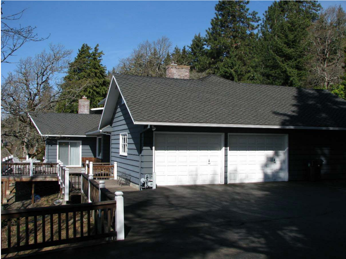
Figure 9. Van Alstine House east and south elevations, looking west.
