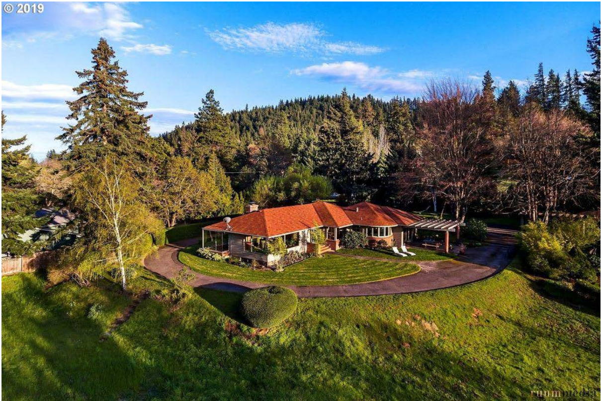
View: North and west elevations, viewing southeast. (Zillow.com)
