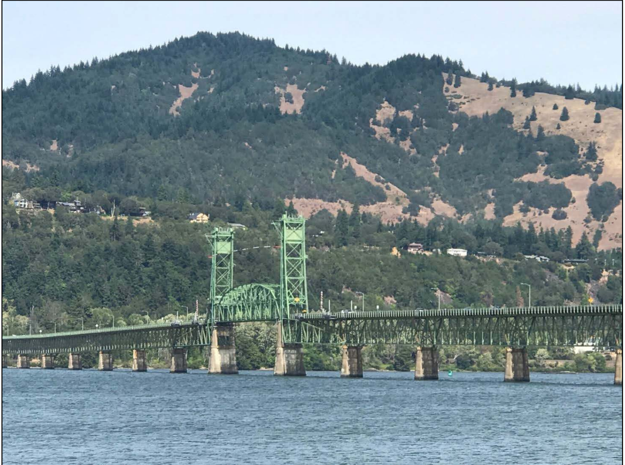
Figure 1. Detail of lift span looking east, 2019. (Source: Lys Opp-Beckman).
