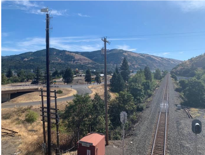
OR&N segment within APE, just east of Hood River, viewing east (AECOM 2020)
