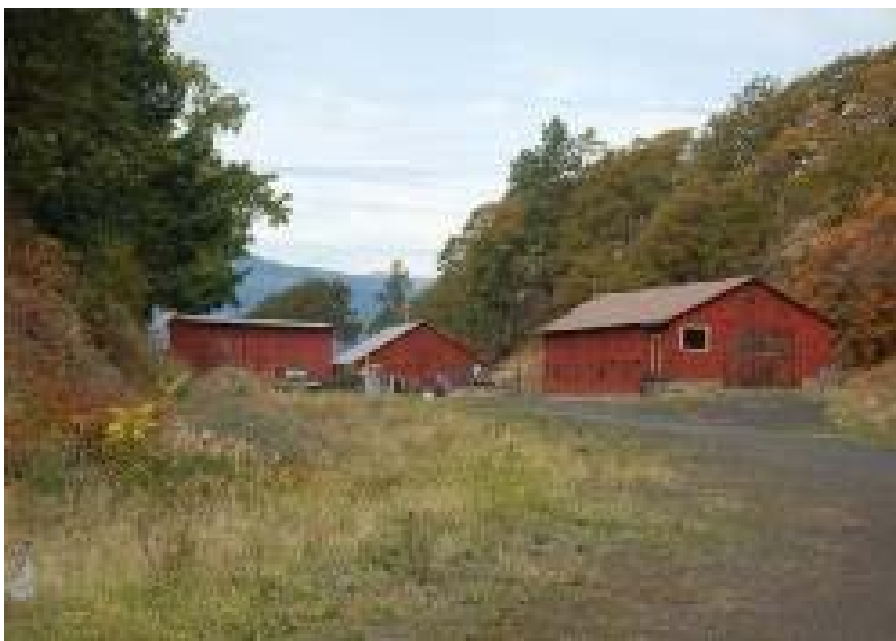
Figure 3. Photograph of 2495 Old Columbia River Drive, looking north towards Hood River Bridge.
