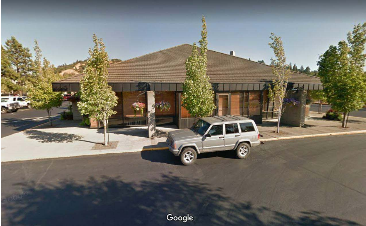
View: Northwest elevation, viewing southeast (Google Earth Pro 2020).
