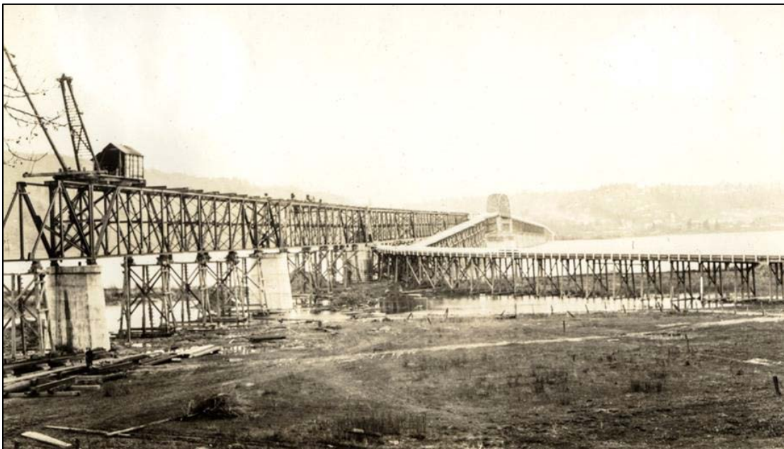
Figure 6. Construction of new north approach, on the left, 1938. Photo Credit: historichoodriver.com .
