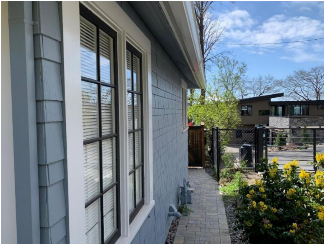
Figure 6-4. 267 SE Oak Street west elevation, looking southwest towards Hood River Bridge.
