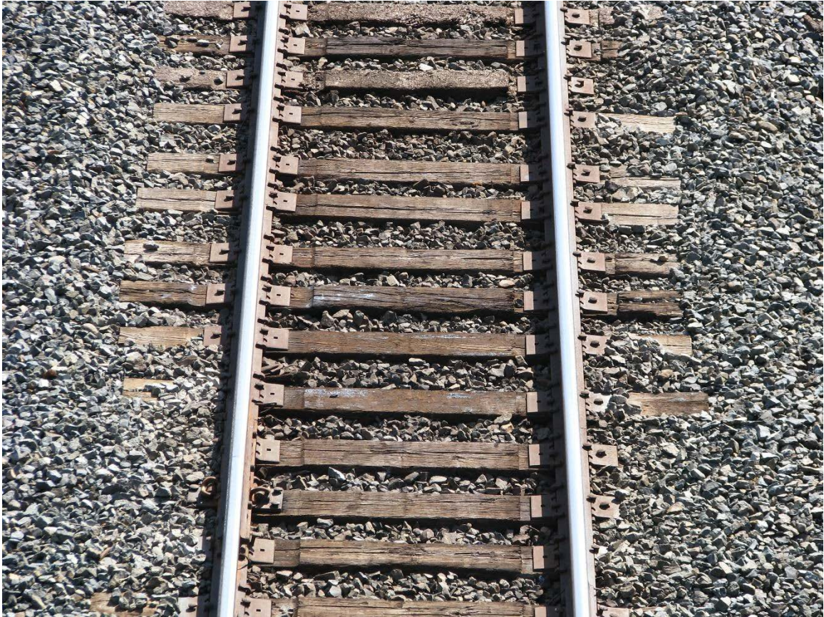
Figure 4. OR&N segment, view from above.
