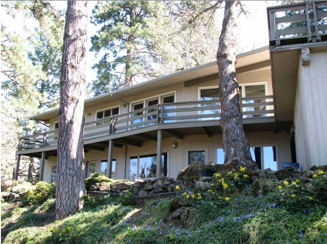
View: Northwest elevation, viewing northeast.
