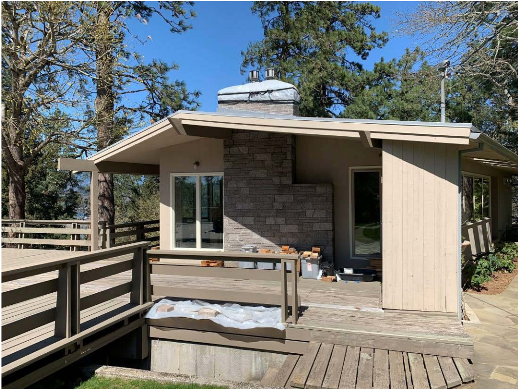
View: Southwest elevation, viewing northeast.
