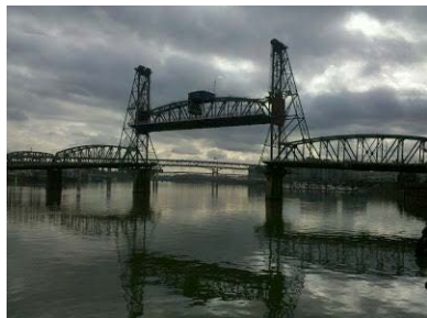
Hawthorne Bridge (courtesy of MBI Motors)
