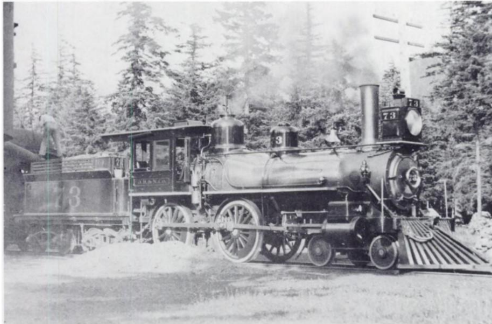
OR&N No. 4, "The Spokane Flyer," which ran daily in 1900, is pulled by OR&N No. 73 (4-4-0) and is stopping at Bridal Veil, Oregon to take on water.
