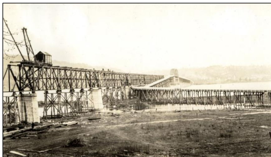
Figure 4-22. Construction of new north approach, on the left, 1938 (Historic Hood River).
