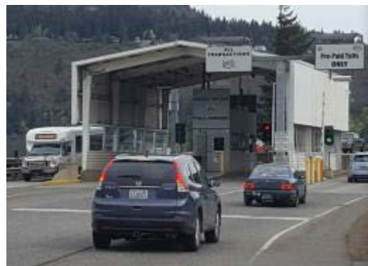
Figure 2. Detail view of tollbooth, looking north, 2018. (Source: WSP USA, Inc.).
