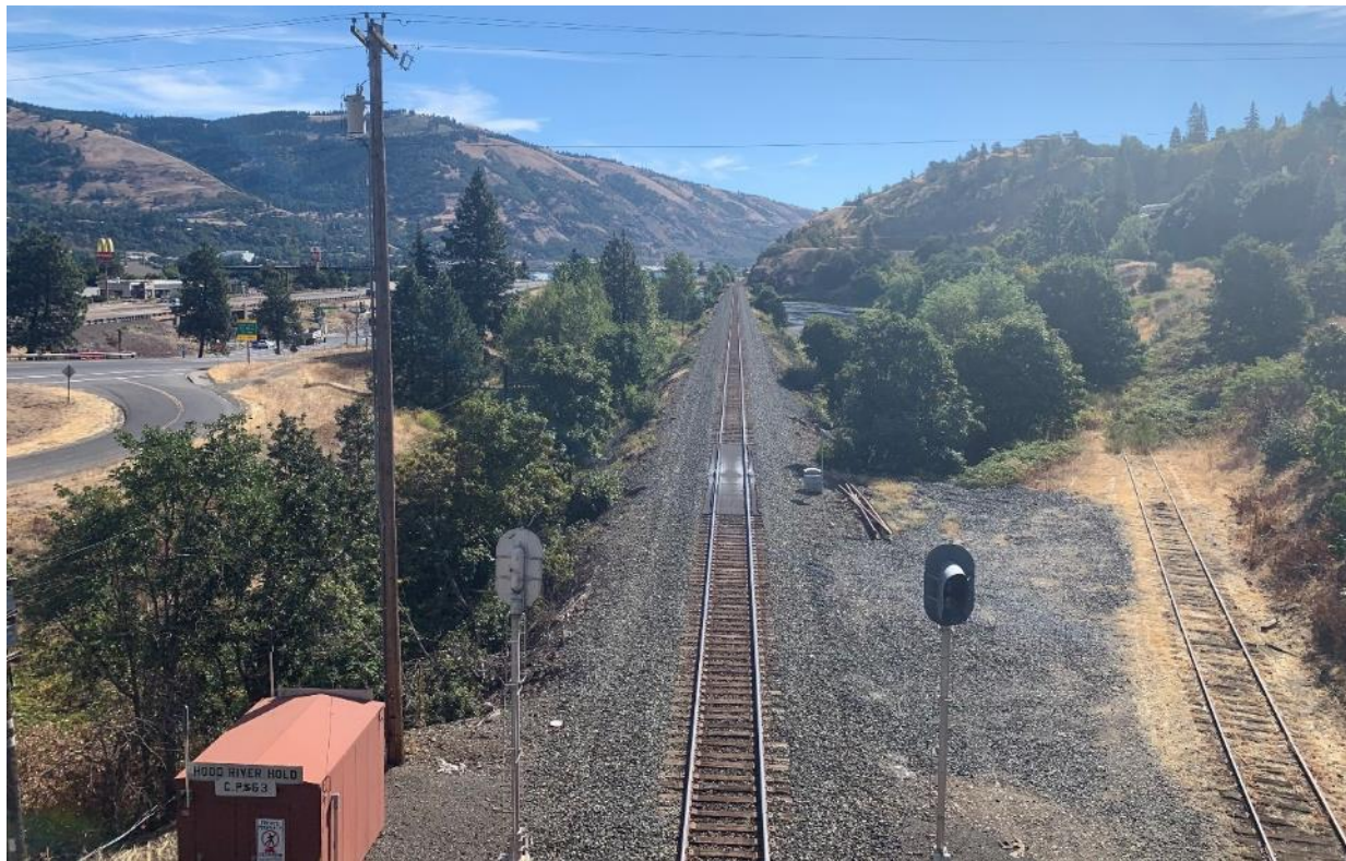
Figure 6-16. Photograph of OR&N segment in Hood River, Oregon (looking east)
