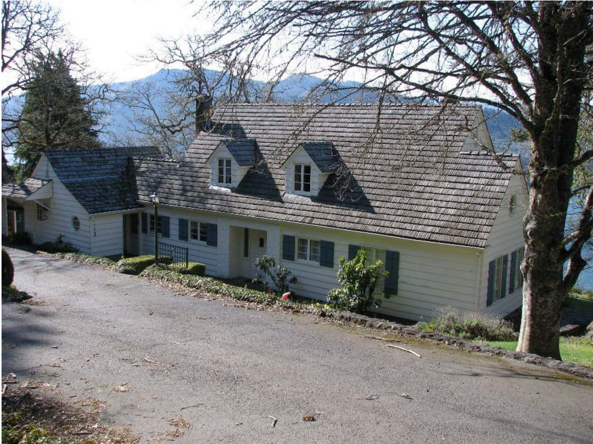
Figure 3. Photograph of 447 W Jewett Boulevard, looking southeast towards Hood River Bridge.
