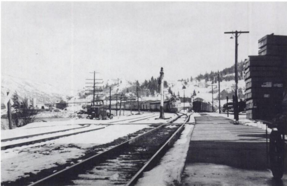
The westbound "Idahoan" arrives in Hood River on a clear, wintery day in 1947. Notice the cardboard boxes stacked on the handcar (right) which contain live baby chickens being shipped to Portland. The spout close to the track (center) furnishes water for the remaining steam engines. Also notice the 1929 Model A Ford Tudor.
