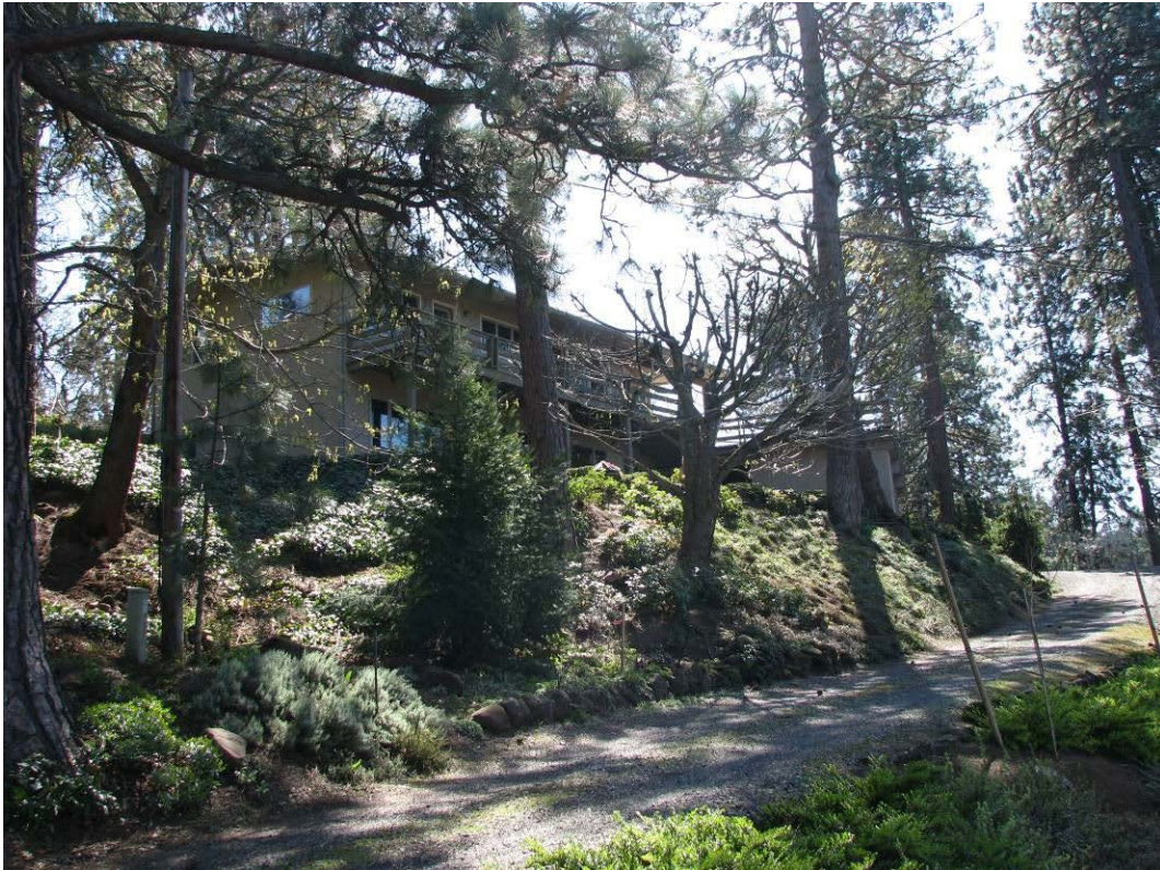
View: Northwest and northeast elevations, viewing south.
