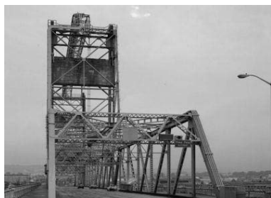
Murray Morgan Bridge (courtesy of the Library of Congress/HAER by Bridgehunter.com)
