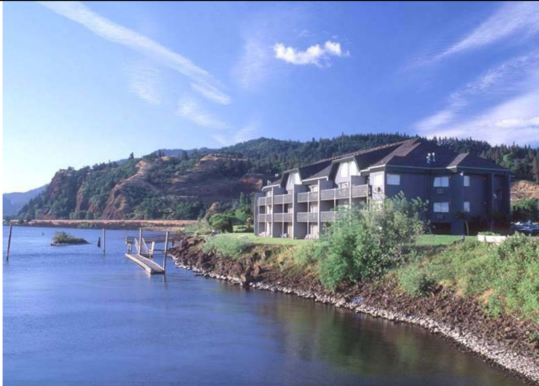
View: West wing, facing east (Hood River Inn 2020a)
