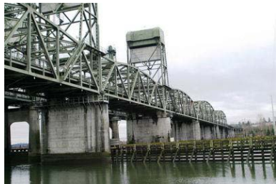
Snohomish River Bridge (SB) (courtesy of bridgehunter.com)
