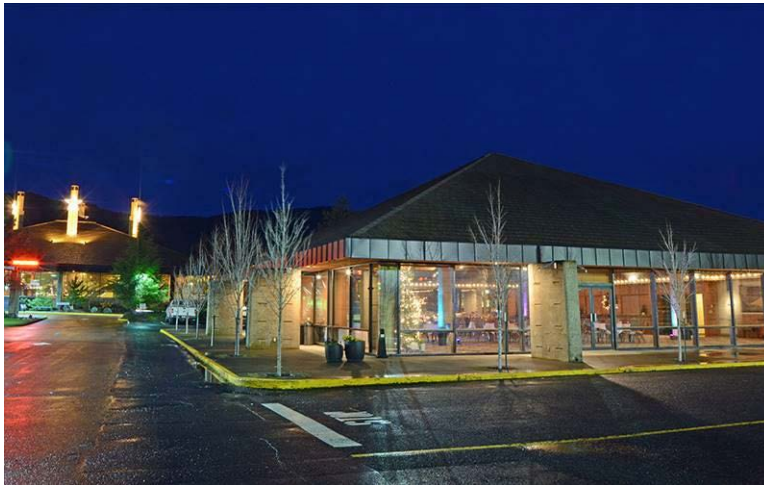
Southwest Elevation, Viewing Northeast (Photo Credit: HoodRiverInn.com)
