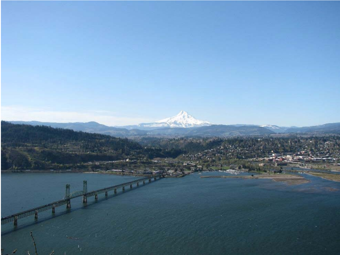
Figure 9. Photograph from 447 W Jewett Boulevard looking southeast towards Hood River Bridge.
