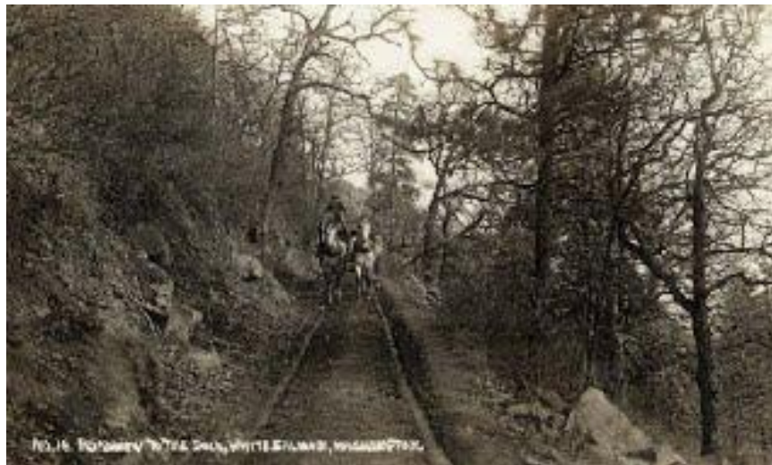
Figure 4-6. Construction of Dock Grade Road, connecting the dock to the town of White Salmon (Gorge Heritage Museum 2020).
