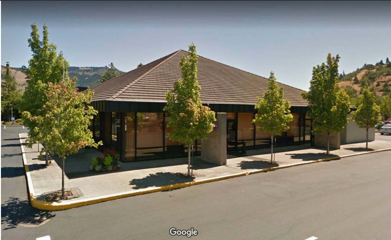
View: Southwest elevation, viewing east (Google Earth Pro 2020).
