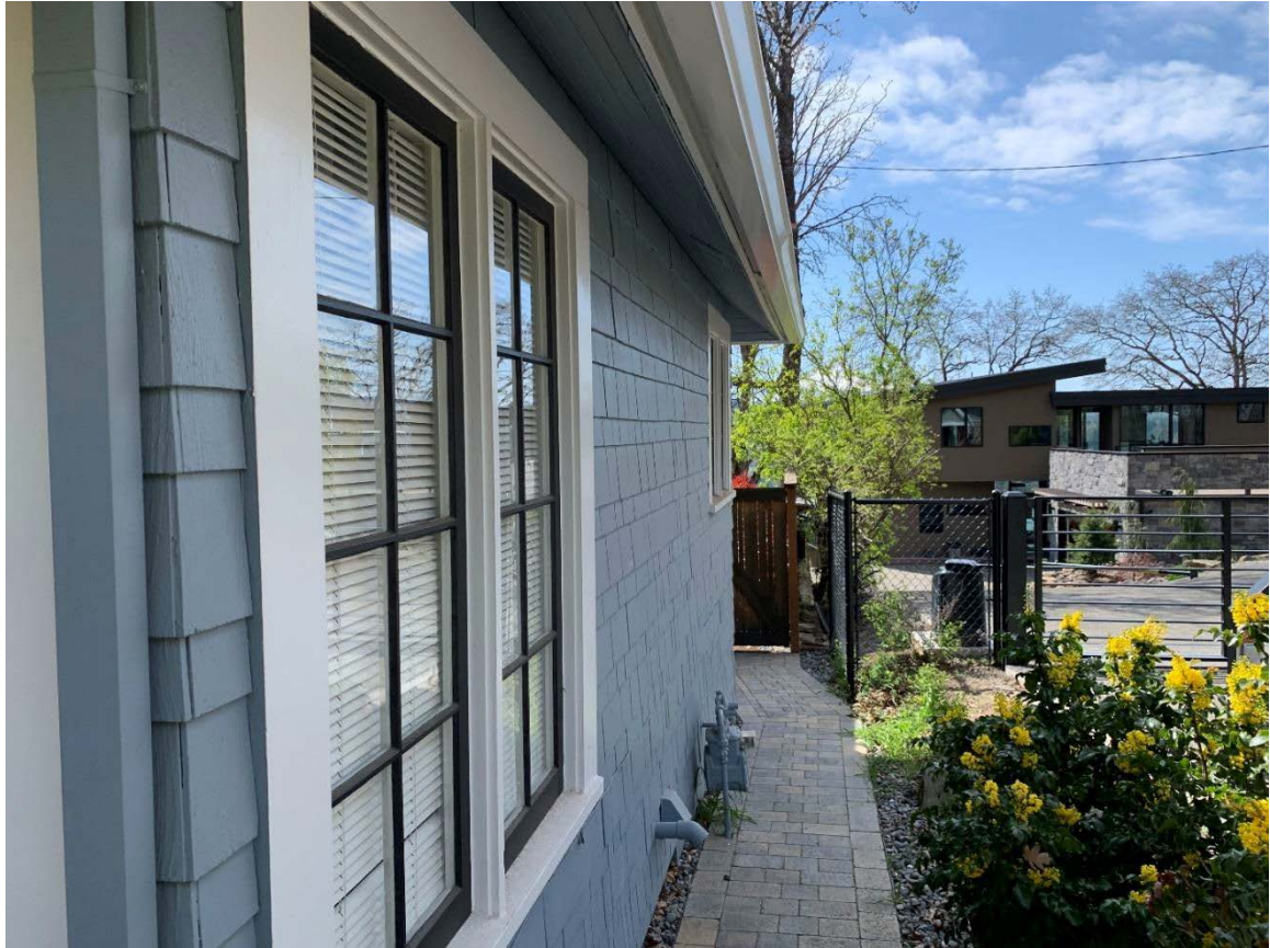
Figure 8. 267 SE Oak Street west elevation, looking southwest towards Hood River Bridge.
