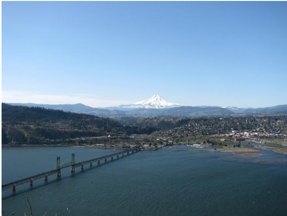
Figure 6-12. Photograph from 447 W Jewett Boulevard looking southeast towards Hood River Bridge
