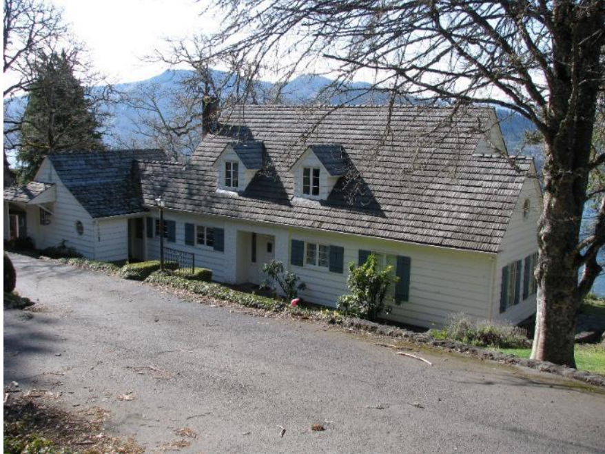
Figure 6-11. Colonial Revival-style residence at 447 W Jewett Boulevard (1940) in White Salmon, Washington.
