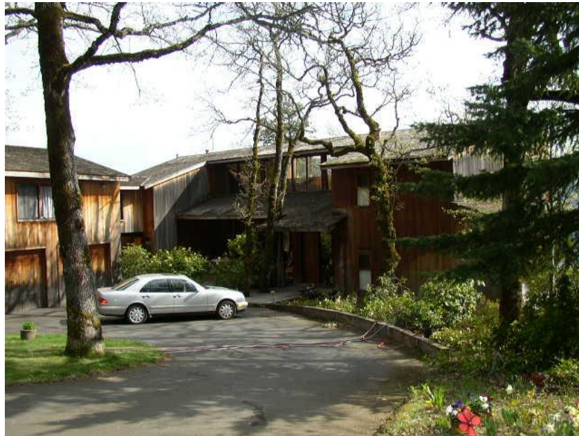
Figure 6-8. Northwest Regional residence at 345 W Jewett Boulevard, White Salmon, Washington
