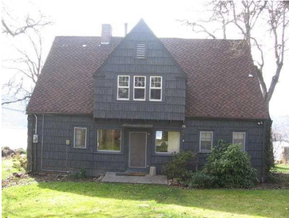
Photograph 1_301 SE Oak Street.jpg
