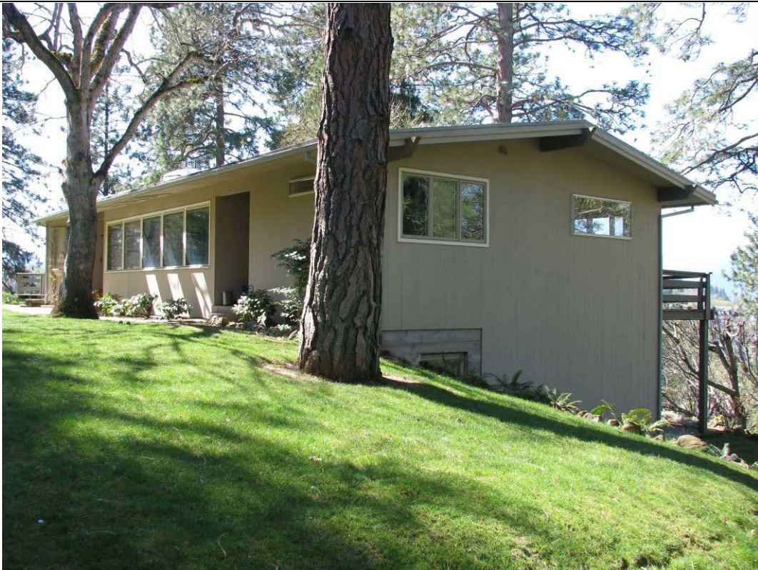
View: Northeast and southeast elevations, viewing west.
